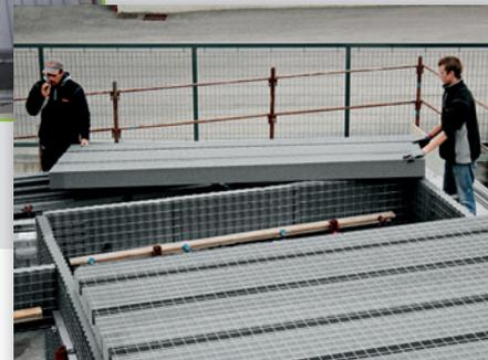
**INSTALLATION OF THE FLOOR PANEL WITH THE LATTICE GIRDER****8**
